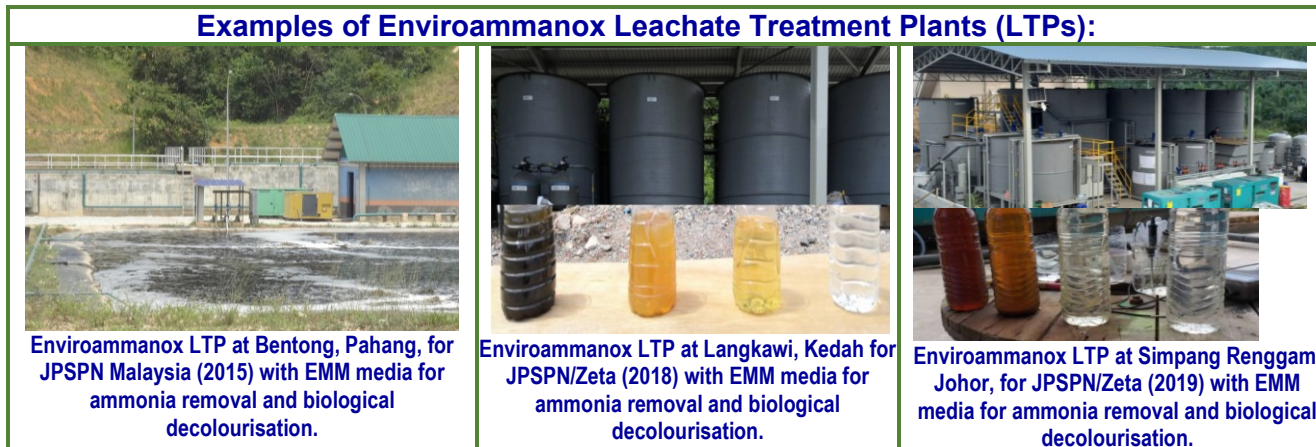
Dark leachate biologically decolourised without any chemical usage at Bentong LTP
